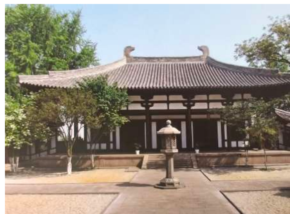
Figure 4. The large roof with ornamental projection of Jianzhen Memorial Hall, Yangzhou, Jiangsu
