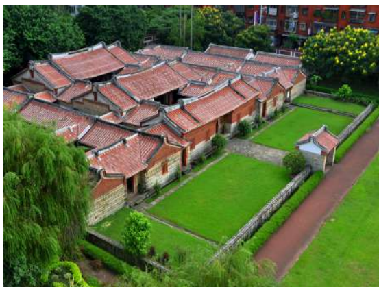
Figure 3. The "horseback spine" roof of Luchou Lee Family Residence, New Taipei City, Taiwan
